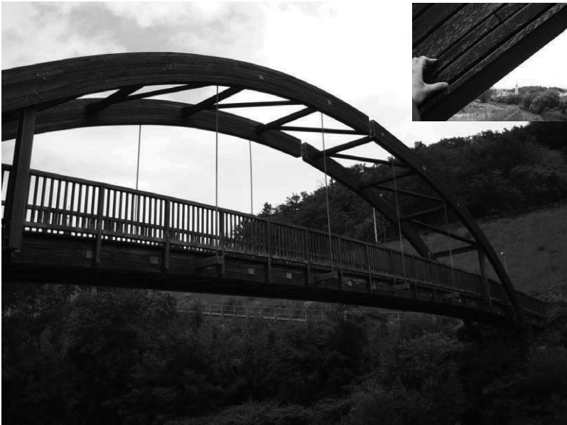
Figure 2: Bolt-laminated Ekki bridge at Finowfurt, Germany.
