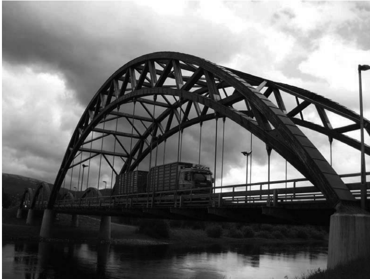
Figure 3. 70m span bridge at Tynset, Norway; one of the longest timber bridges in the world designed for full highway loading. To achieve the 100 year design life the glulam members were treated with CCA before laminating and creosote after laminating and the upper surfaces were also protected with copper caps.
