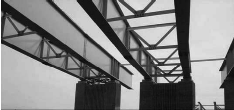
Figure 1. Pairs of braced beams awaiting deck slab construction
