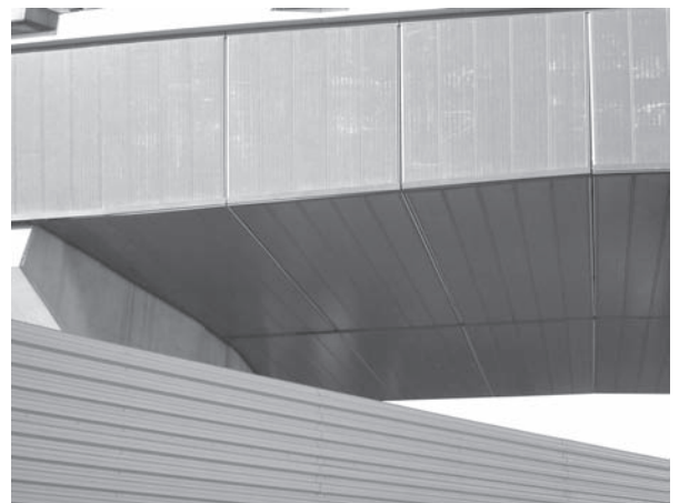
Fig. 43.3 Photograph of the enclosure on the approach span of the Dartford River Bridge (QE2) where it passes over the CTRL (before the train rails were laid) (Courtesy of AECOM).
