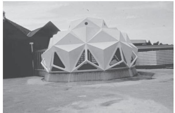
Fig. 43.1 The 'all-polymer composite' classroom of the primary school, Thornton Clevelys, Lancashire, UK.
