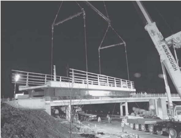
Fig. 43.5 Craning in the 100-tonne FRP deck onto the supports of the bridge over the M6 (Courtesy of Mouchel).
