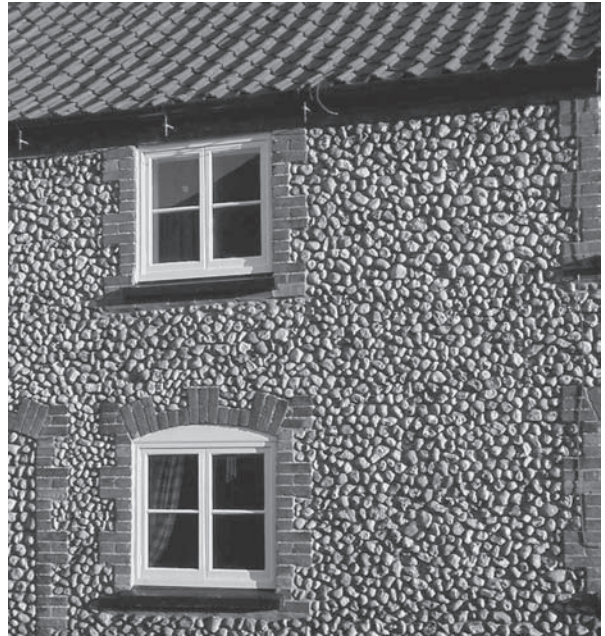
Fig. 37.7 Well-conserved flint-work masonry in Norfolk.
