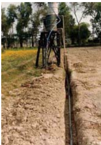
Fig. 7.6 Main and lateral laying
