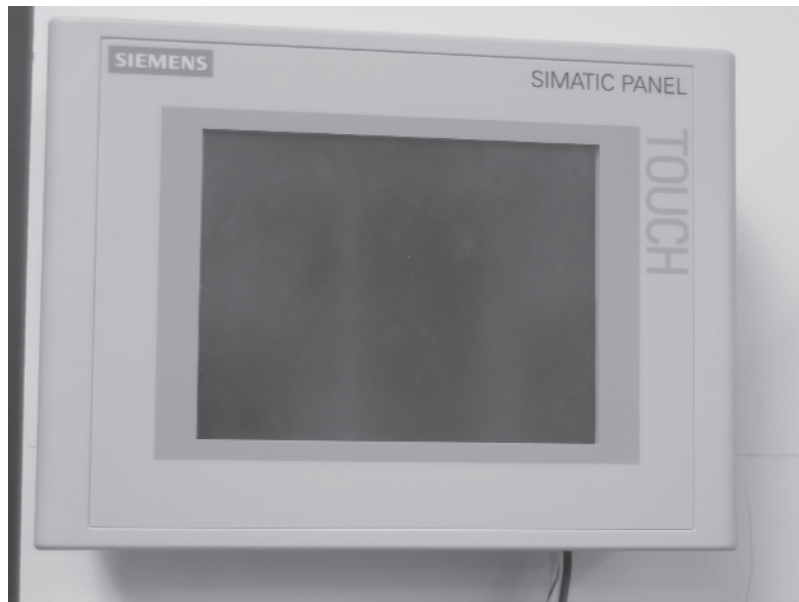
FIGURE 9–9 Human machine interface (HMI) screen to interact with control systems.
