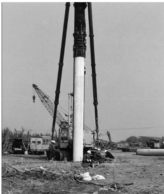
Figure 8.2 Driving of a precast concrete pile with a single-acting Delmag D-100-13 diesel hammer in Jiayi, Taiwan. (Courtesy of An-Bin Huang, Hsinchu, Taiwan.)
