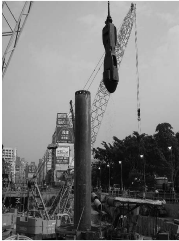
Figure 8.26 Field operation of an oscillator rig used to insert casing and a hammer grab. (Courtesy of An-Bin Huang, Hsinchu, Taiwan.)
