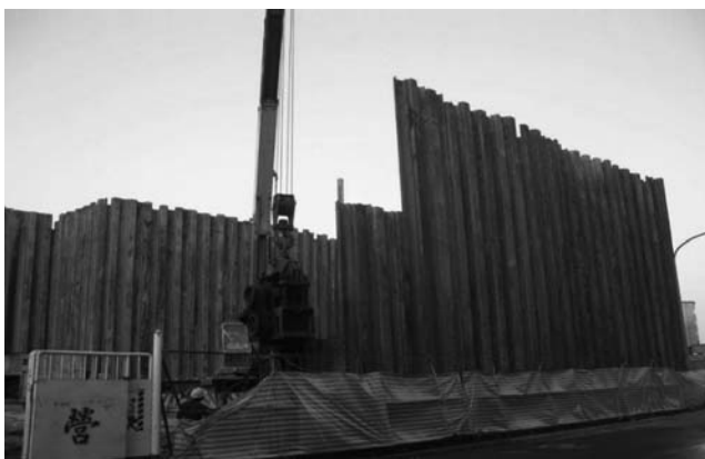
Figure 5.22 Field installation of a sheet pile wall. (Courtesy of Trinity Foundation Engineering Consultants, Co. Ltd., Taipei, Taiwan.)
