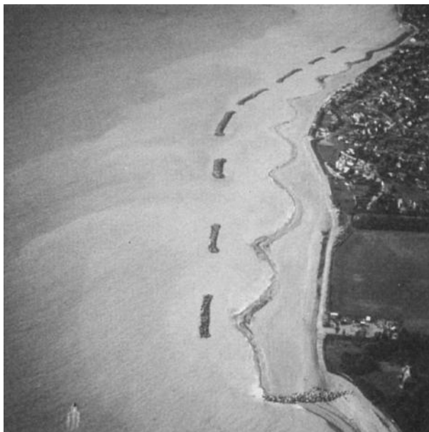
FIGURE 16.5 Aerial view of the Elmer offshore breakwater scheme.
