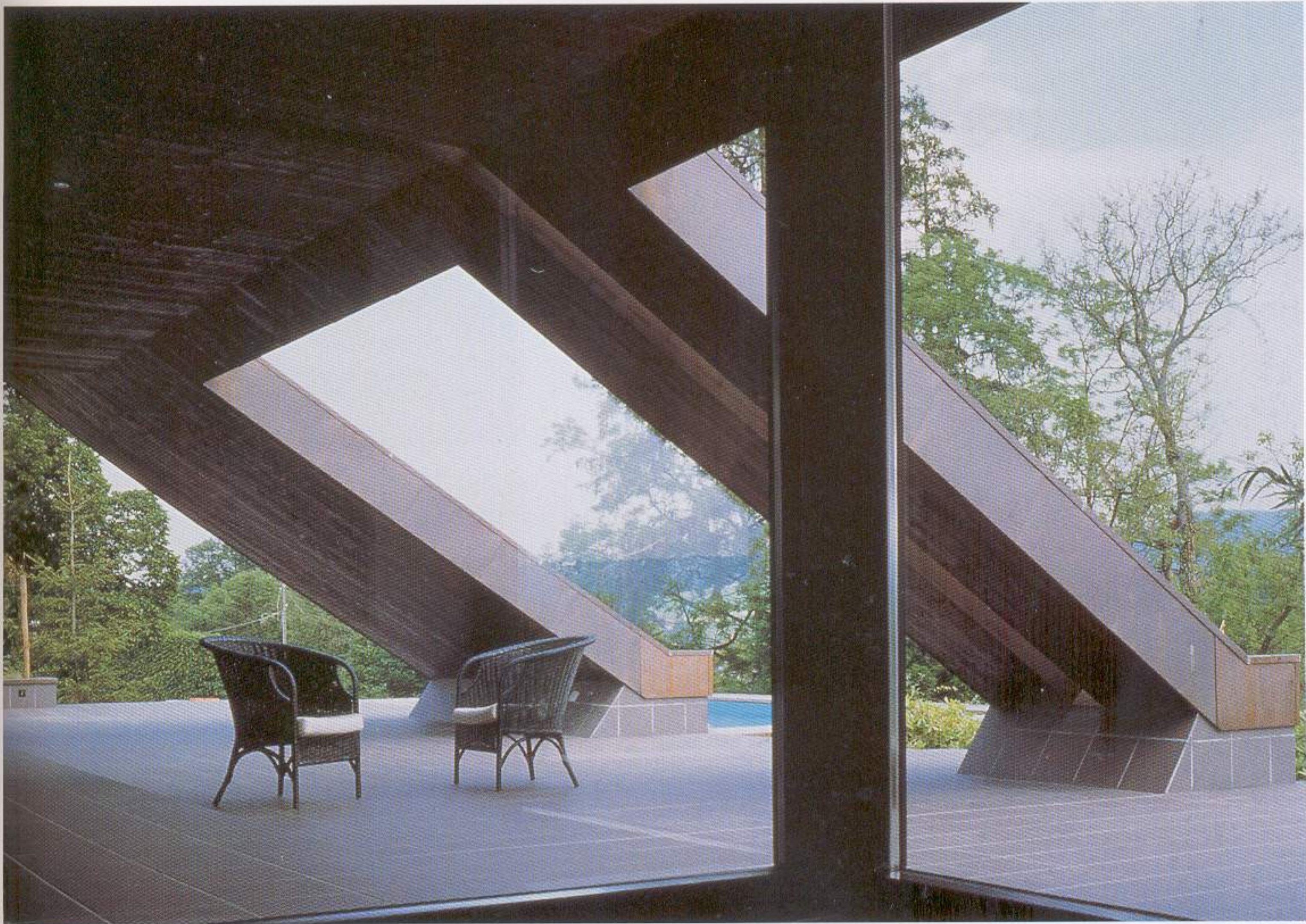
Inside the patio showing the cutouts in the roof that slope to the ground.
