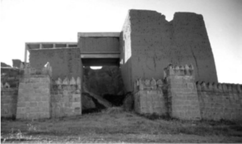
FIGURE 19-1. The restored Adad Gate at Nineveh. One of the fifteen gates of the city.
