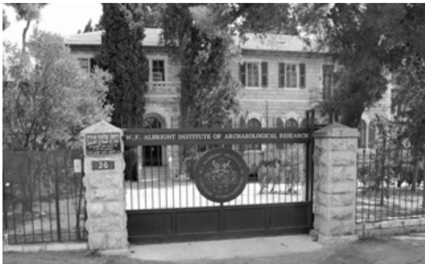
FIGURE 5-1. The “Albright,” as the Albright Institute for Archaeological Research is affectionately known. This Jerusalem building was constructed as the original home of the American Schools of Oriental Research in the 1920s. It is now named for an early director, the influential archaeologist William F. Albright.
