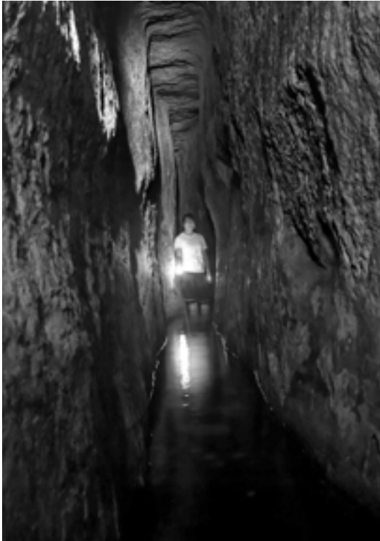
FIGURE 15-2. The narrow tunnel dug during King Hezekiah's reign to bring water from the Gihon Spring just outside the city walls into Jerusalem proper.
