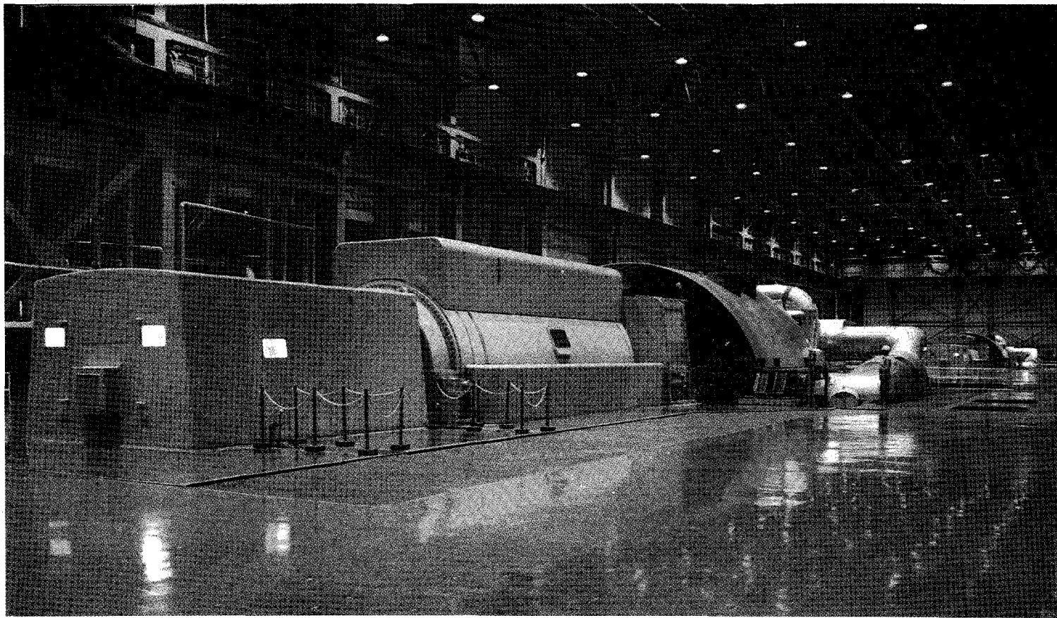
500 MW steam turbine-generator sets at 2000 MW Singrauli Super Thermal Power Station of NTPC—supplied and executed by BHEL, India (Courtesy: NTPC and BHEL, India)
