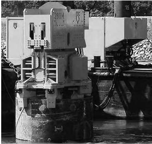
Figure 3.16 Driving a pile casing with a PVE 200 m free hanging vibrator.
