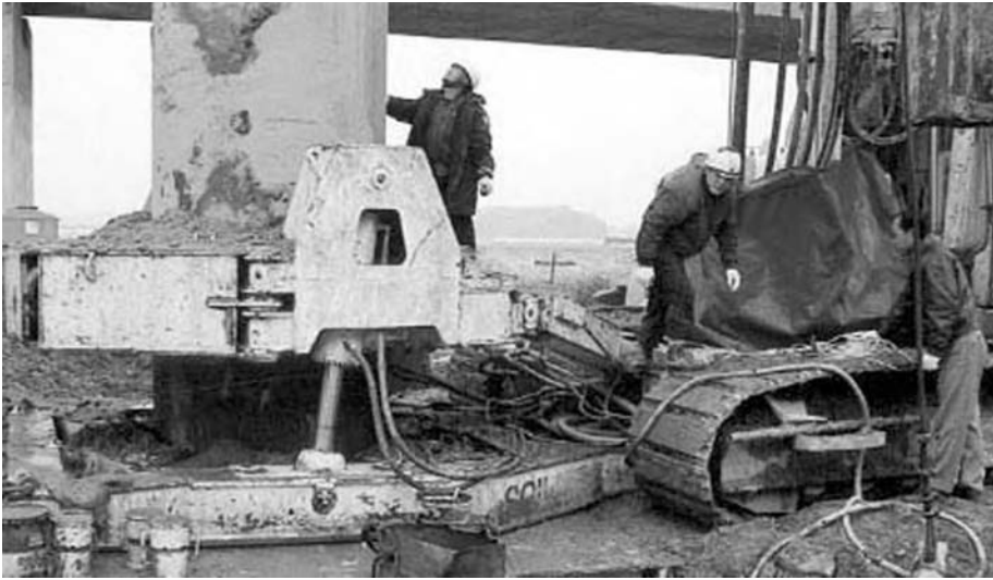
Figure 3.31 Soilmec casing oscillator.
