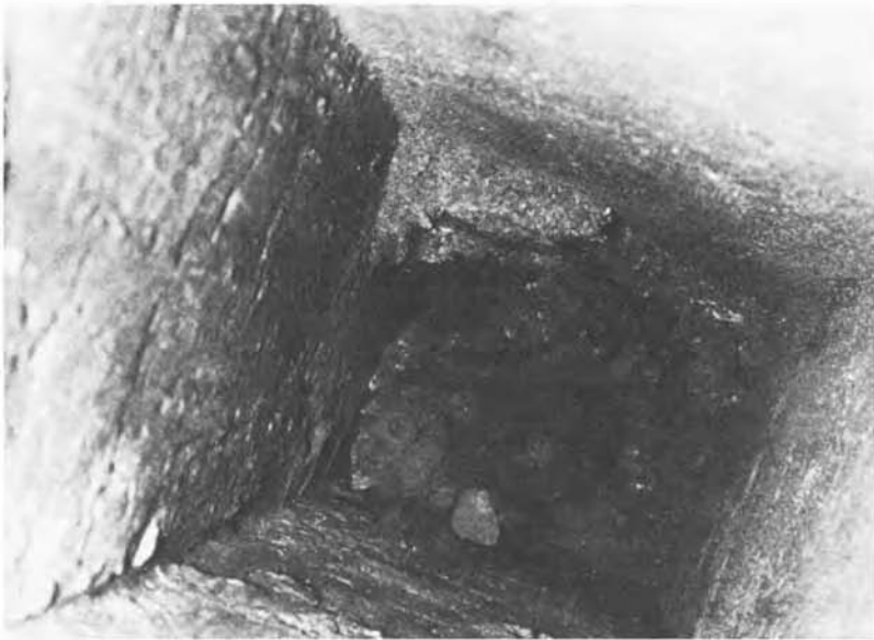
Figure 10.1 Decay of timber piles above groundwater level (Crown copyright reserved) (a) Cavities left by complete decay of piles and timber capping sills (b) View down cavity left in clay after complete decay of timber pile.
