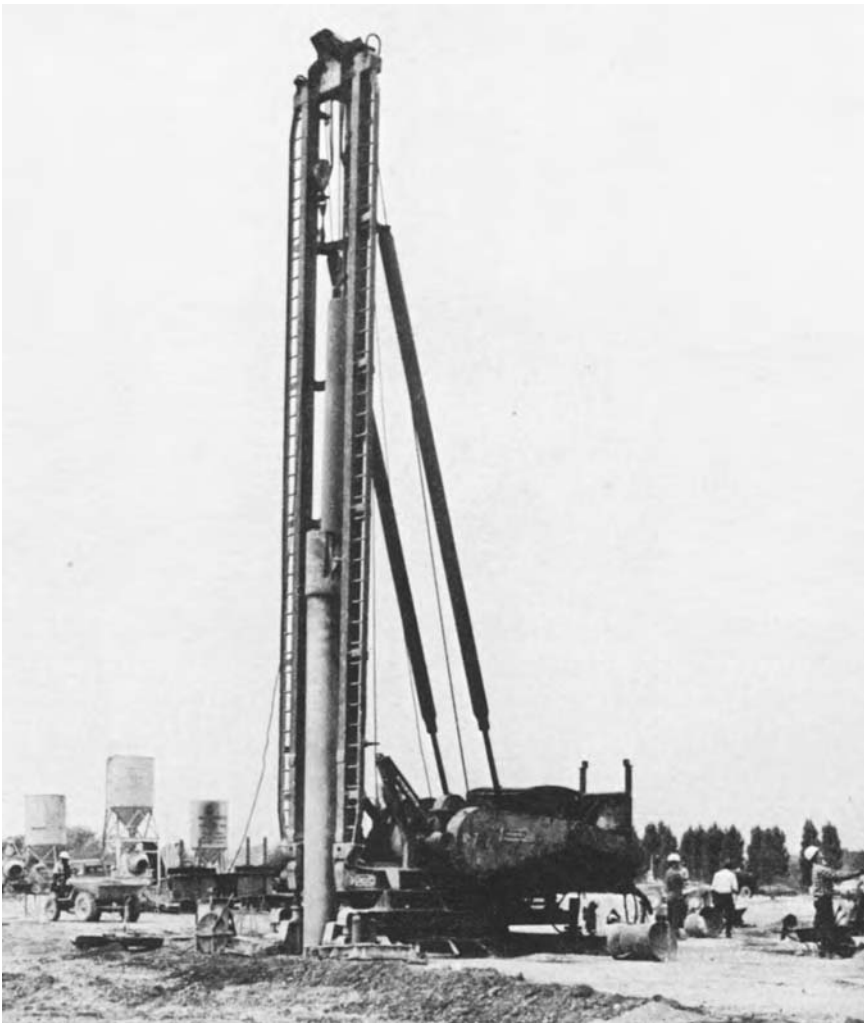
Figure 3.23 Franki pile-driving rig.
