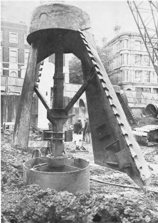
Figure 3.30 Top-hinged under-reaming bucket.
