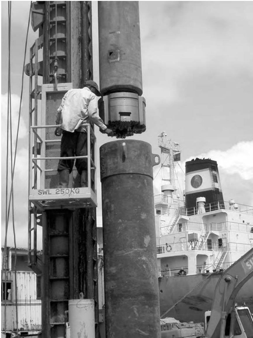
Figure 3.32 Numa hammer with extending under-reaming drill bit for simultaneously drilling and inserting casing (courtesy Numa Hammers).
