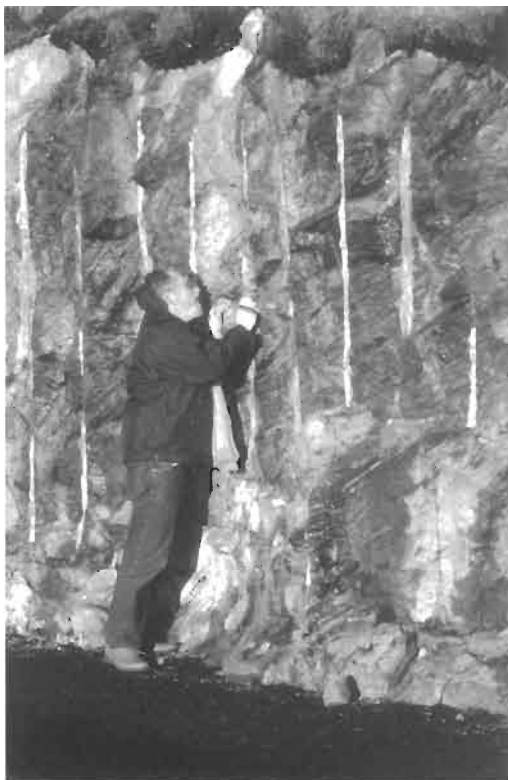
Figure 15.16 A static pre-split formed using expanding grout (Isle of Lewis, Scotland).
