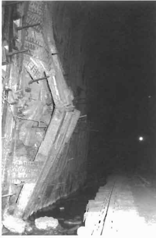
Figure 1.6 Heavily supported tunnel excavated by blasting.
