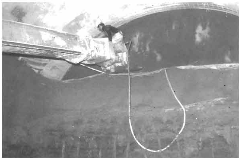
Figure 16.9 Construction of the Bochum metro in Germany.
