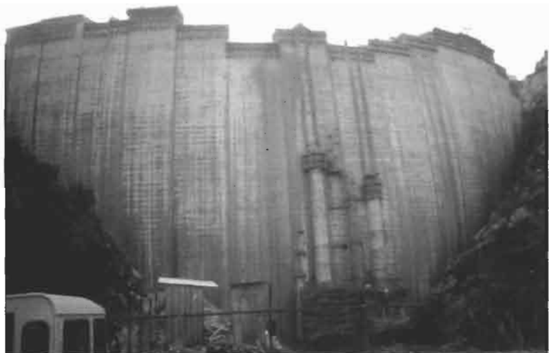
Figure 1.9 Large dam in Portugal.
