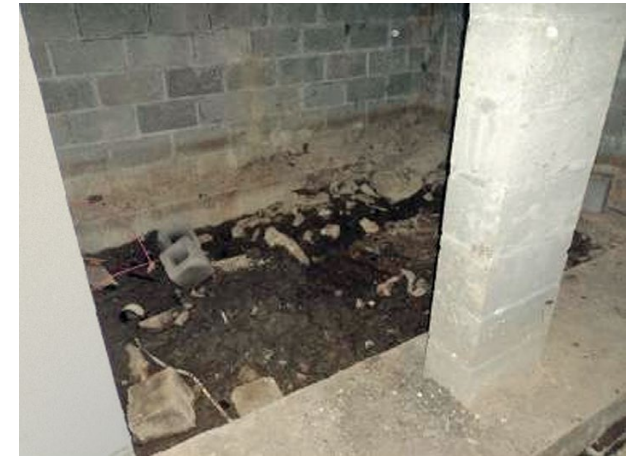
New Foundation at Rosa Keller Public Library, Broadmoor Historic District, New Orleans (2011)
