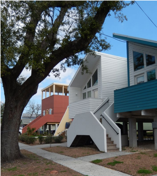
Make it Right Duplex House by Hitoshi Abe Atelier, Lower 9th Ward, New Orleans (2014)
