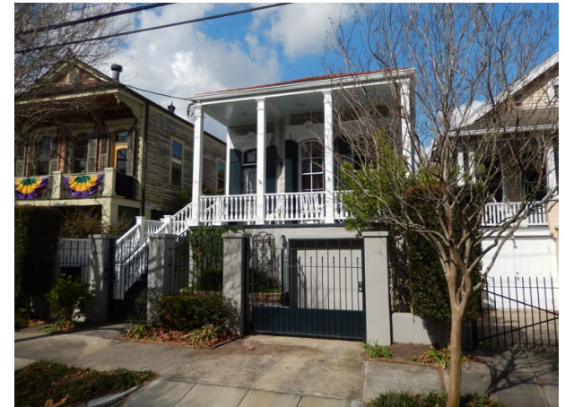
Adjoining property considerations- type, scale, location and patten of block create neighborhood character, Bywater Historic District (above) and Esplanade Ridge Historic District (below), New Orleans (2014)
