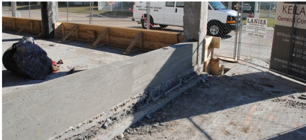
Concrete flood barrier integrated into the existing structure under renovation (2011)
