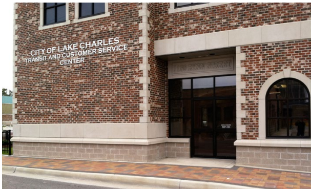
Exterior of building following renovation (2014)
