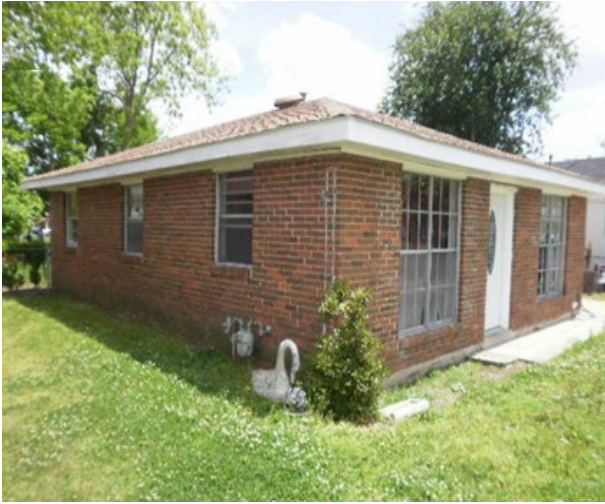
Mid-century home, slab-on-grade, prior to elevation, Harvey. Source: Roubion Inc. ( www.roubionshoring.com )
