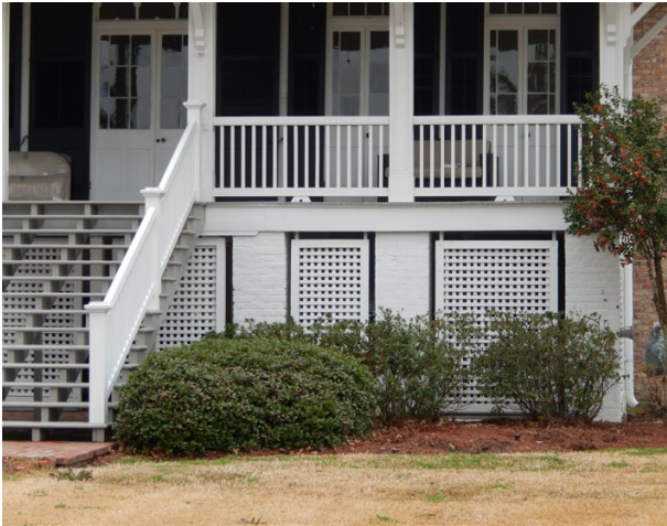
Architectural screening for large areas should complement the features of an existing facade within a new sub-story zone, Mandeville Historic District (2014)
