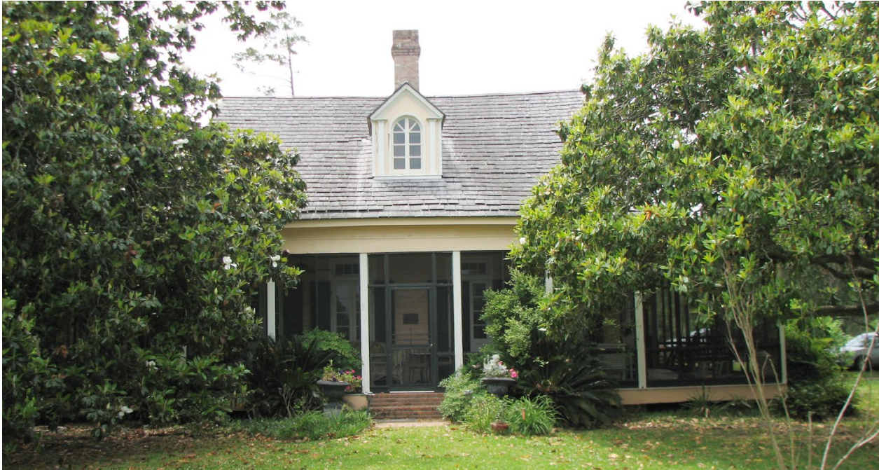
Francois Cousin House, Prior to Elevation, St. Tammany Parish
