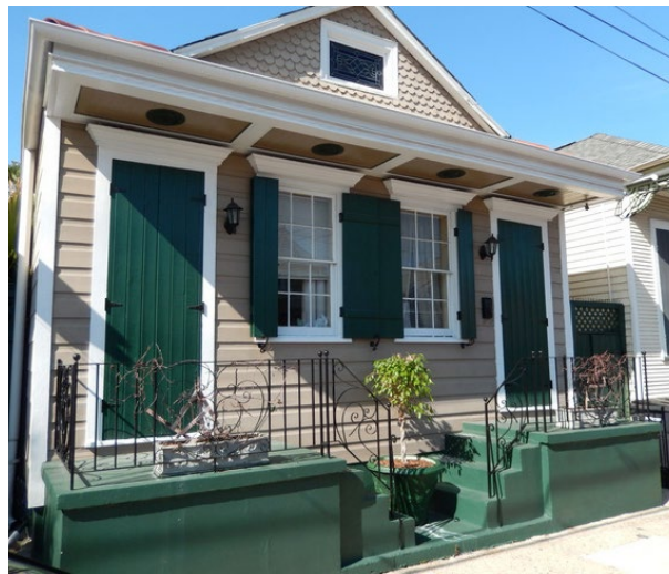
Split Stair Examples, New Orleans (2014)
