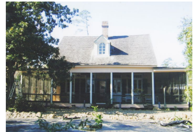
Site Preparation and Clearing Underway
