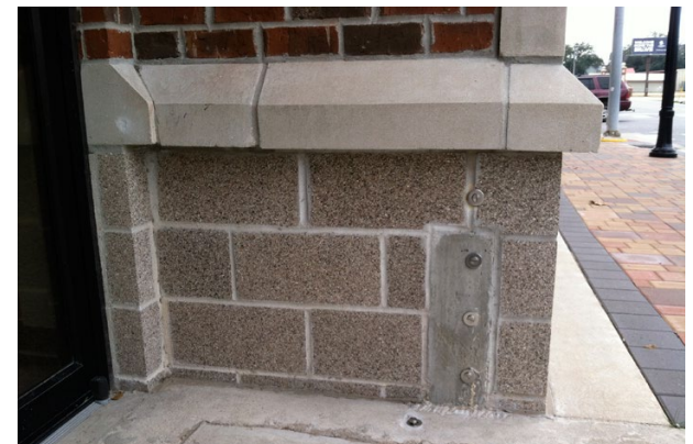
Exterior of building following renovation (2014)
