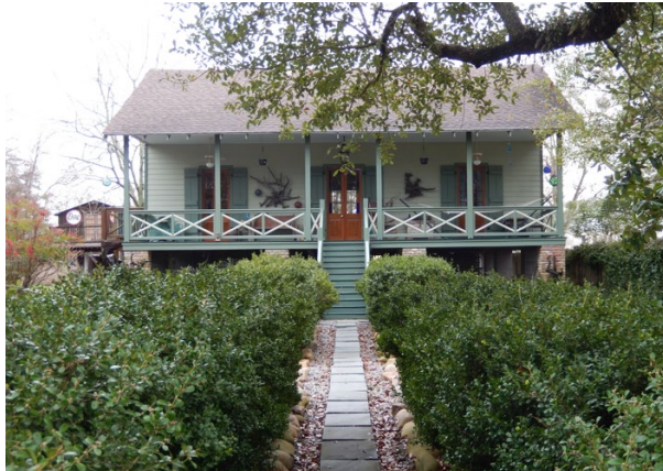
Landscape screening strategies can provide an effective means to minimize the visual impacts of elevation, Mandeville Historic District (2014)
