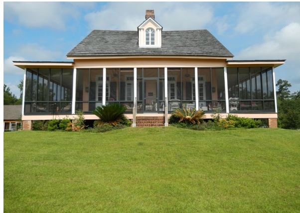
Francois Cousin House, St. Tammany Parish, pictured in 2014 after being raised on an elevated foundation, surrounded/ masked by an earthen berm to protect it from flooding
