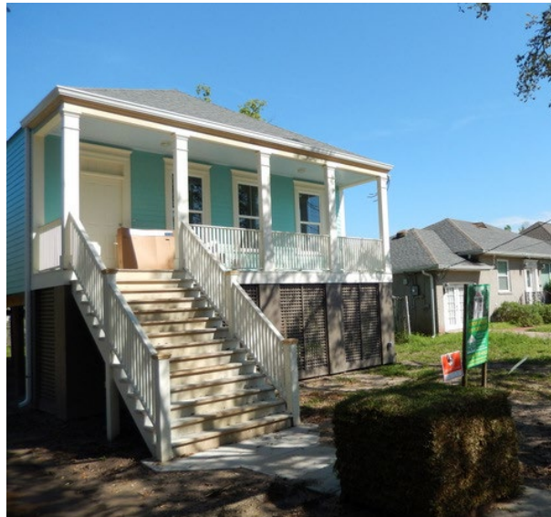
Build Now elevated home, Fillmore Neighborhood, New Orleans (2014)
