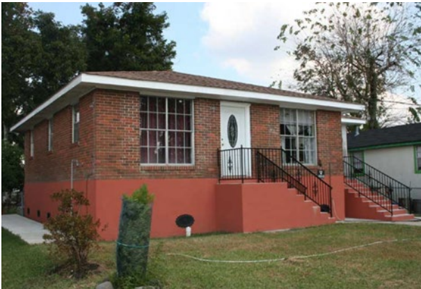
Mid-century home, slab-on-grade, post- elevation, Harvey. Source: Roubion Inc. ( www.roubionshoring.com )
