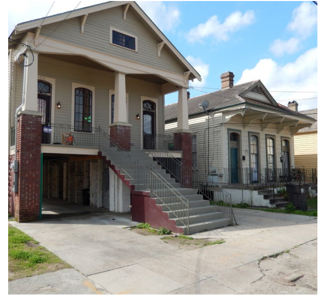
Adjoining properties in the Holycross neighborhood, New Orleans, illustrate the challenges of contrasting elevations, Holycross Historic District (2014)
