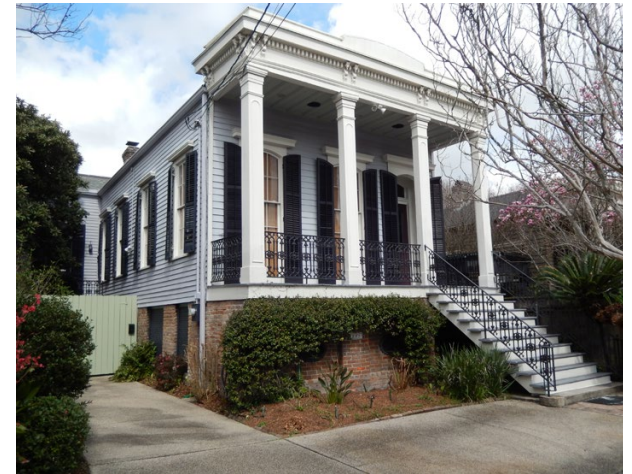
These Guidelines illustrate principles to help preserve the historic elements of homes located in historic districts. Shown here is a raised 3-Bay Shotgun house in the Lower Garden District, New Orleans (2014)
