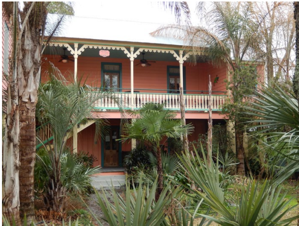
An exterior set of weather-protected stairs is partially concealed beneath the gallery along the side wing (2014)
