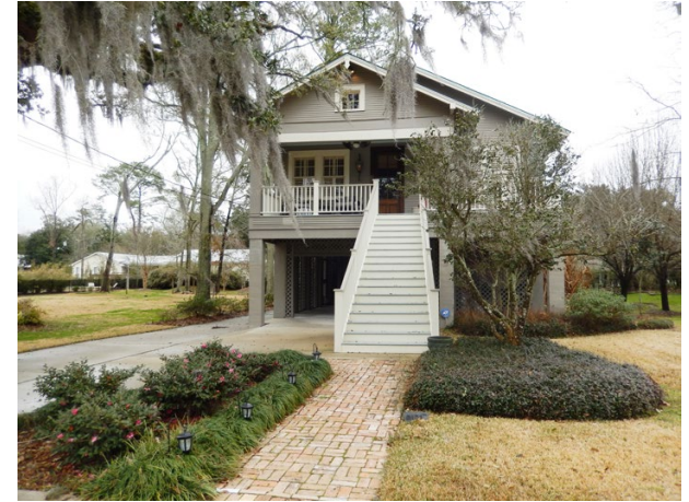
Driveways, parking areas and walkways can have significant influence on the appropriate elevation option, Mandeville Historic District (2014)
