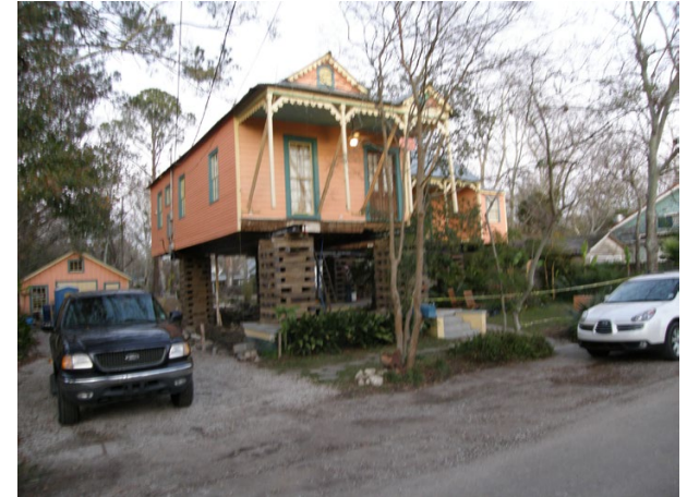
Elevated building supported by cribbing and steel beams (Lynn Mitchell, 2009)
