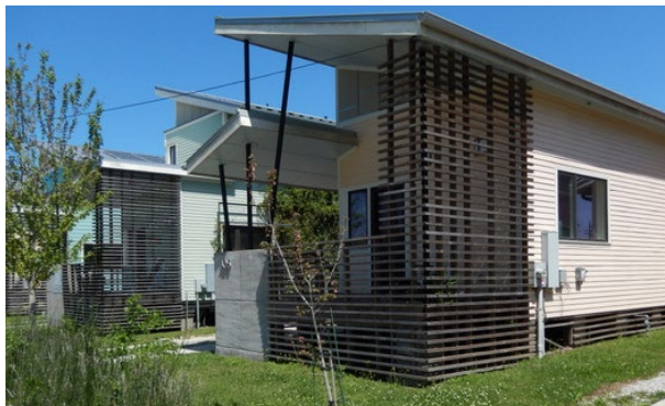
Horizontal wood latticework screens the porch, and its design is repeated at the foundation (2014)
