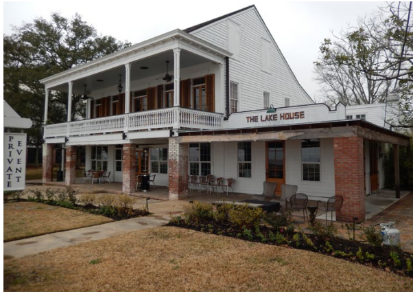
Today a restaurant, the circa 1830's Bechac House in Mandeville represents a pre-Hurricane Katrina elevation of approximately 9 feet above grade and exhibits a repetition of architectural forms, Mandeville Historic District (2014)
