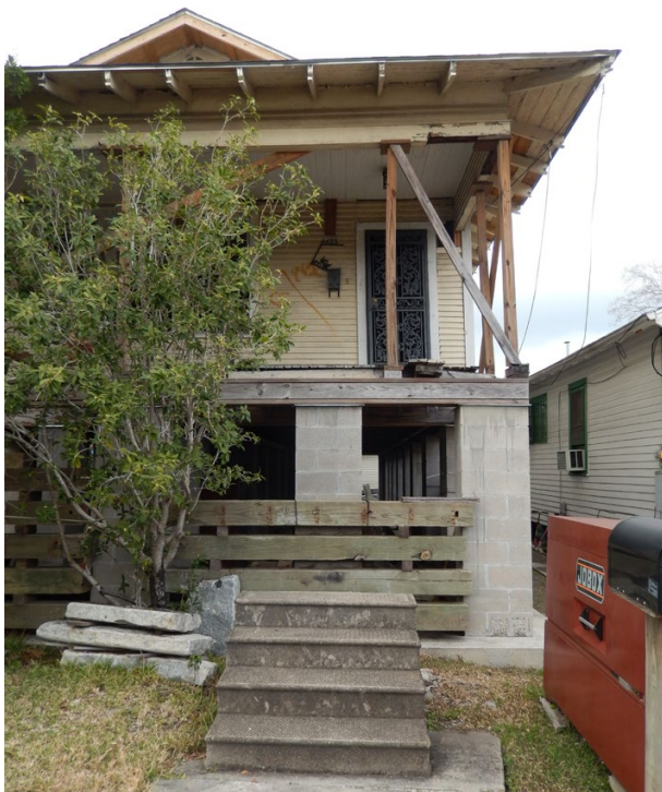
House undergoing elevation in the Broadmoor neighborhood of New Orleans (2014)
