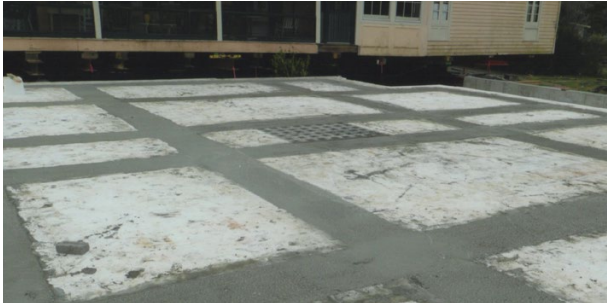
During Construction New Foundation System
