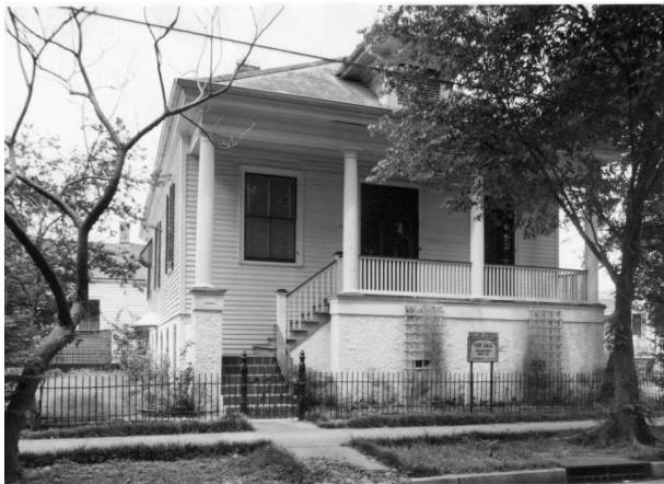
Raised House, 1224 Peniston Street, New Orleans (The Historic New Orleans Collection, used with permission)
