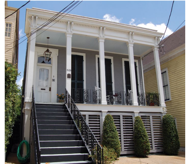
Framed wood louvers can provide effective screening to address elevation changes, Garden District, New Orleans (2012)
