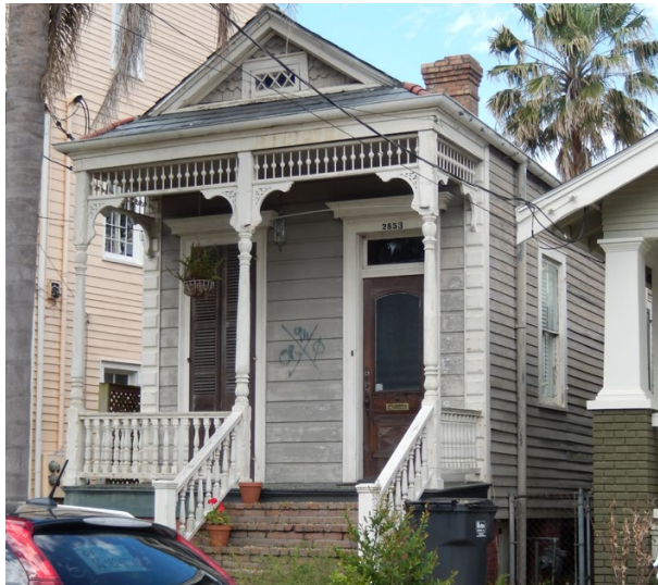
Shotgun House – Façade, New Orleans (2014)
