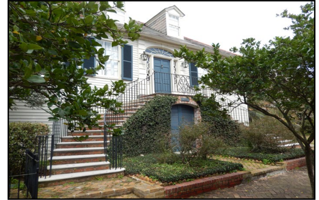
Located in the Lower Garden District, this house depicts a raised first floor living area reached by flanking entry stair, Garden District, New Orleans (2014)
