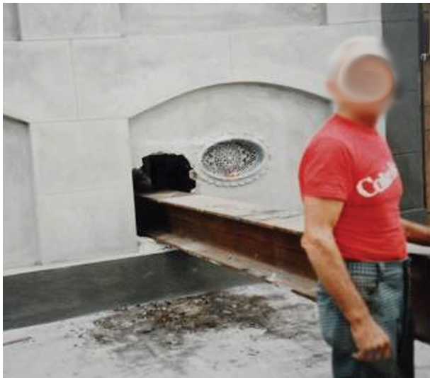
Inserting steel for Rampart Street elevation project, New Orleans (ca. 1980s)
