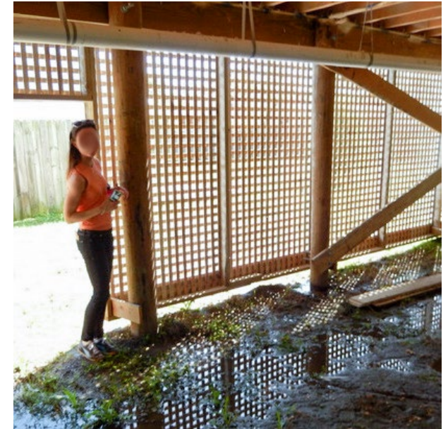
Build Now pile foundation with system of joists, girders, bolts and straps; pilings attach to girders with two three-quarter-inch galvanized steel bolts, and to the floor joists with steel hurricane ties, strengthening the connection between the house and the pilings (2014)
