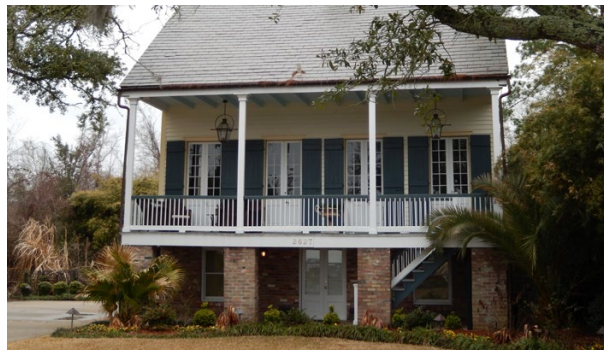
Sub-story elements should coincide with existing vertical references to columns, Mandeville Historic District (2014)
