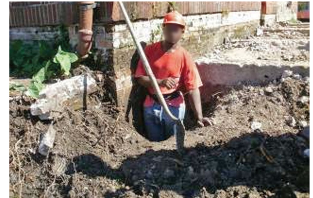
Excavation at Rosa Keller Library, Broadmoor Historic District, New Orleans (2011)
