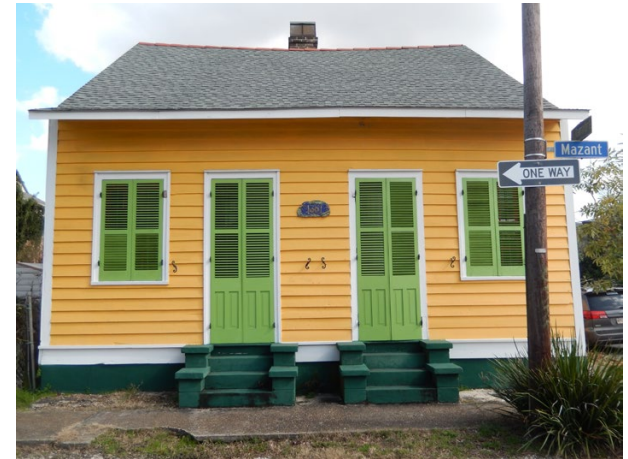
Creole Cottage, Mazant and N. Rampart Streets, New Orleans (2014)
