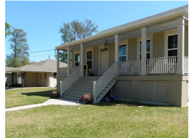
Build Now elevated home, Fillmore Neighborhood, New Orleans (2014)
