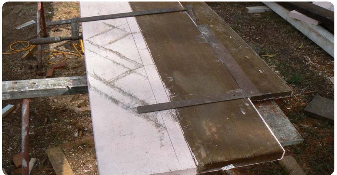
Figure 5.7: Marking out left string.
