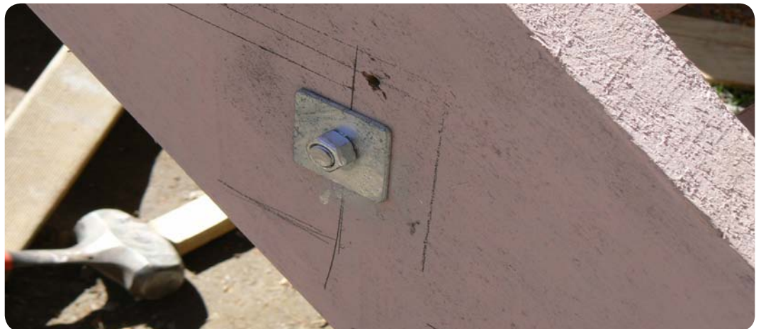
Figure 5.15: Position of step bolt.
