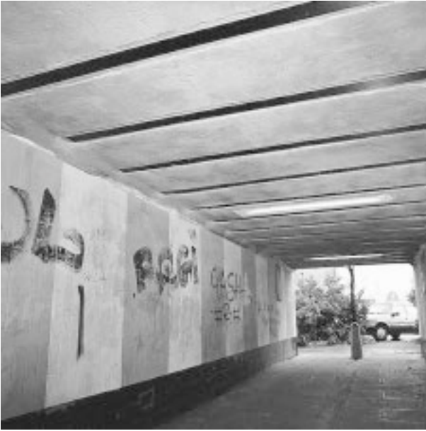
Figure 11.25 View of completed bonding operation, subways, Tyne and Wear.
