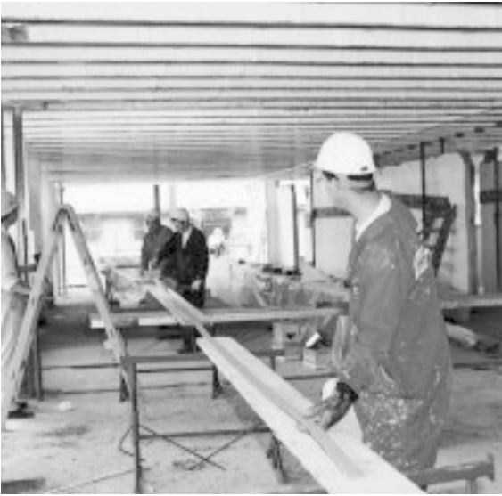
Figure 11.2 Application of adhesive to CarboDur laminate.
