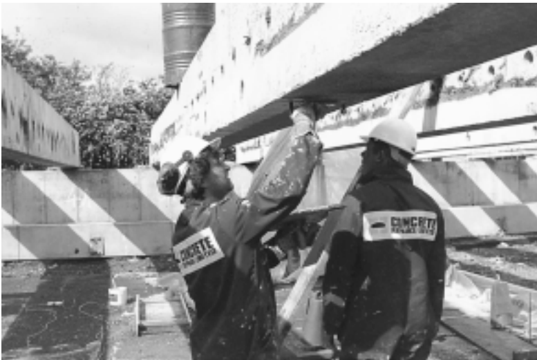
Figure 10.1 Applying epoxy adhesive to prepared concrete surface.
