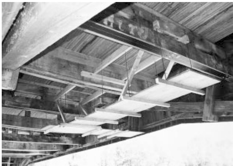
Figure 11.21 View of strengthened cross beams.
