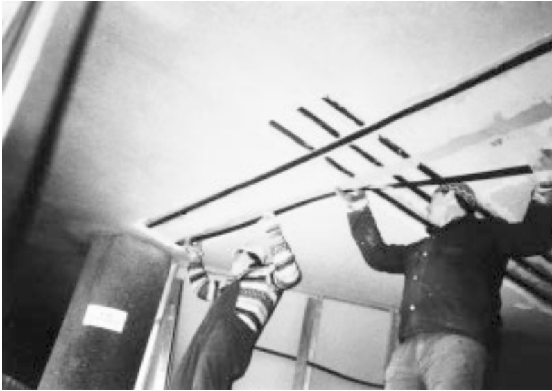
Figure 11.32 Application of CarboDur laminates.
