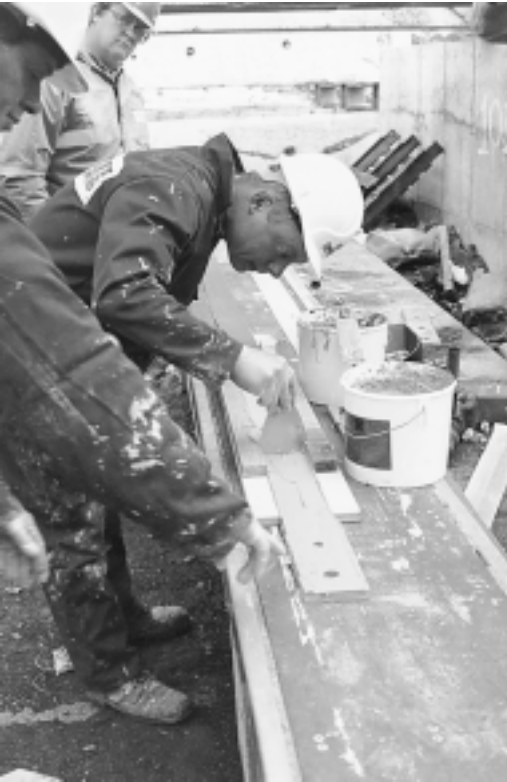
Figure 10.2 Setting dome-shaped spatula into adhesive reservoir prior to application of epoxy adhesive to plate.
