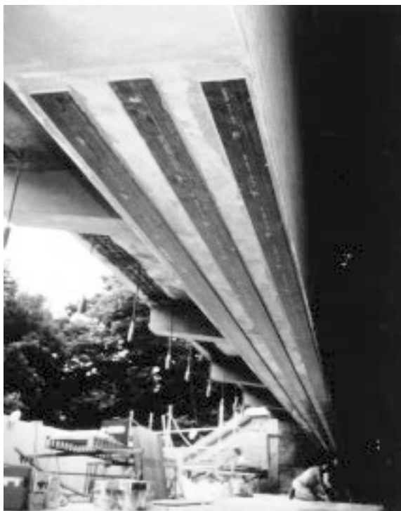
Figure 11.40 View of post-strengthened beam.
