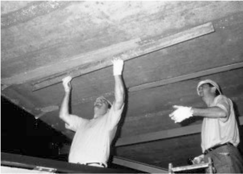
Figure 11.13 Checking the evenness of the reprofiled surface.
