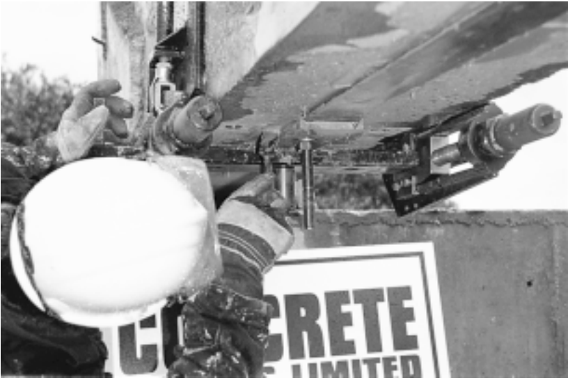
Figure 10.10 Inserting the anchor bolts after applying the required prestress load.
