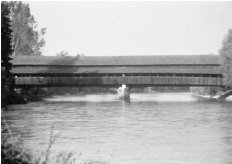
Figure 11.18 General view of wooden bridge, Sins, Switzerland.
