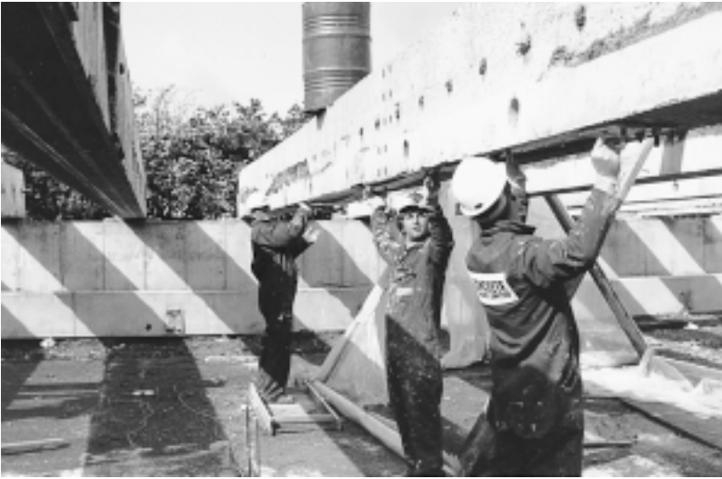
Figure 10.3 Fitting CFRP plate to concrete surface.
