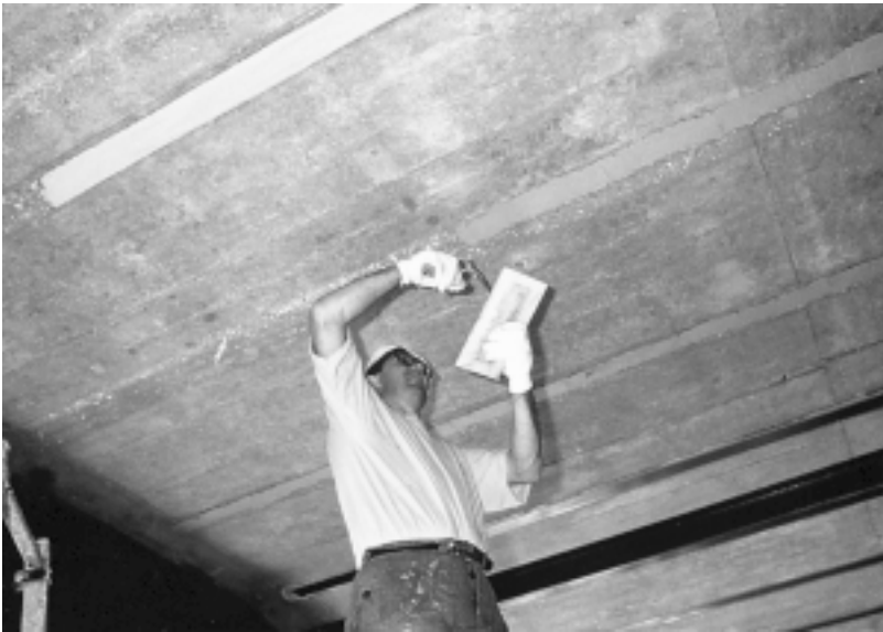
Figure 11.9 Application of the Sikadur epoxy adhesive.
