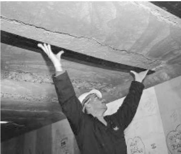
Figure 11.24 Applying CarboDur laminate to underside of underpass, Tyne and Wear.
