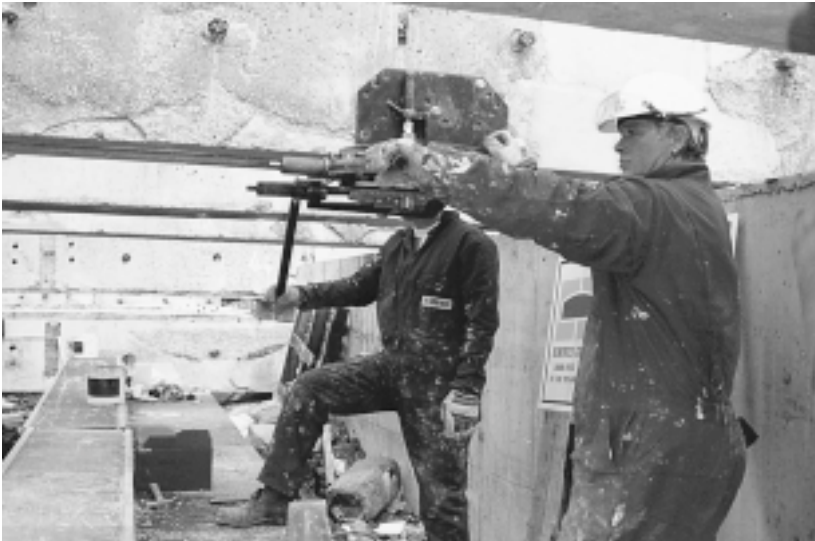
Figure 10.9 Using the twin screw jacks to tension the plate and apply prestressing.
