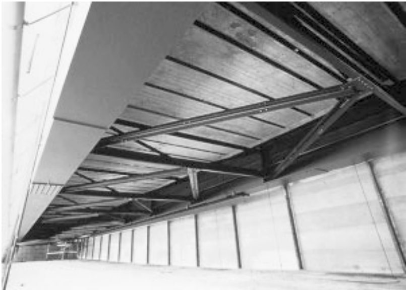
Figure 11.14 Completed strengthening work on Rhine bridge, Oberriet.
