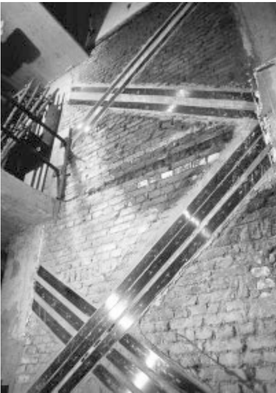
Figure 11.17 URM fire wall strengthened with CarboDur carbon fibre strengthening system.
