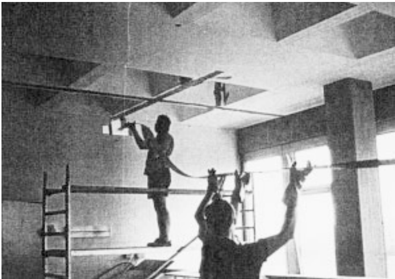
Figure 11.37 Offering CarboDur laminates up to the roof beams, Stuttgart.
