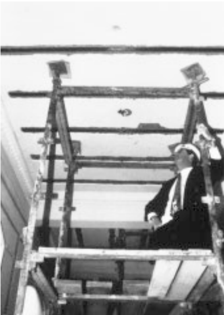
Figure 11.35 View showing plates bonded to structural floor slab substrate.
