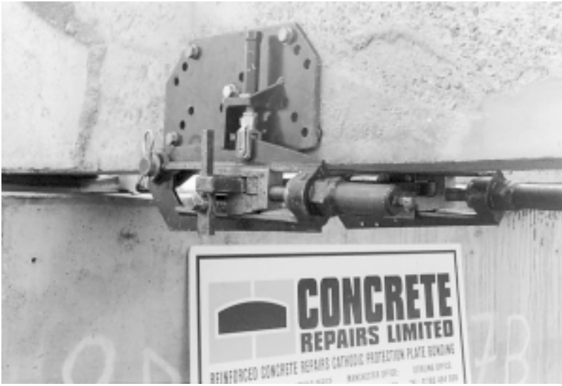
Figure 10.7 Prestressing machine bolted in place to a reinforced concrete beam.
