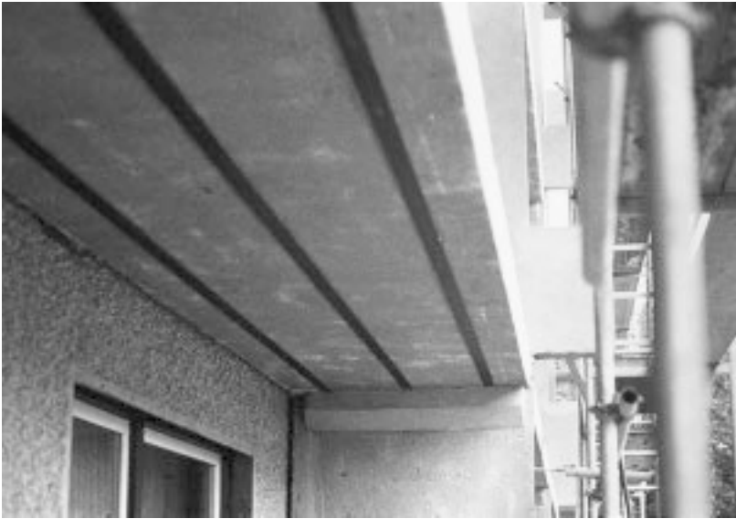
Figure 11.29 Underside of deck showing completed strengthening of balconies, Magdeburg.
