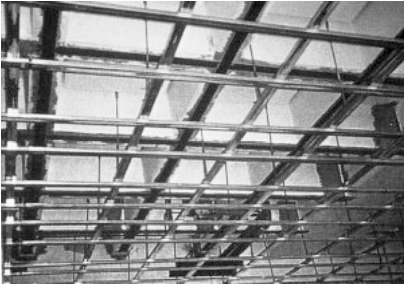
Figure 11.38 The completed project with simple crossover details shown, Stuttgart.
