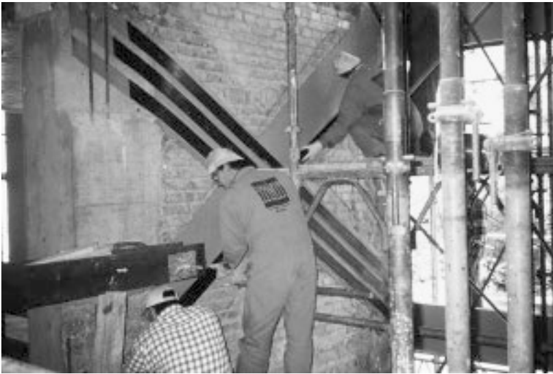
Figure 11.16 Application of the CarboDur plates to the masonry wall.
