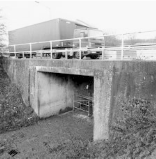
Figure 11.26 General view of the underpass, Great Missenden.
