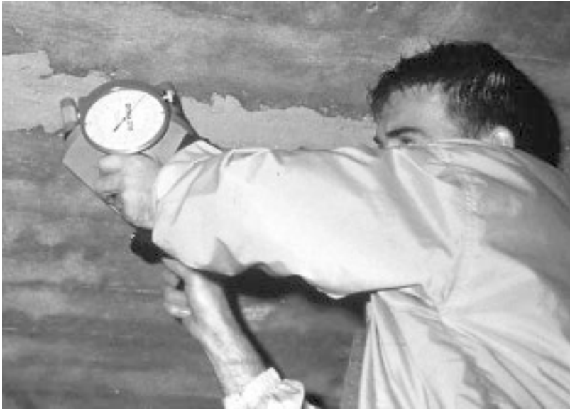
Figure 11.12 Determining the concrete surface preparation by a 'pull-off' test.
