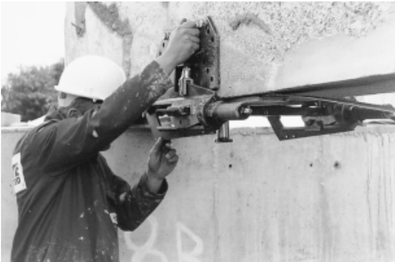
Figure 10.8 Connecting the CFRP plate to the prestressing machine.
