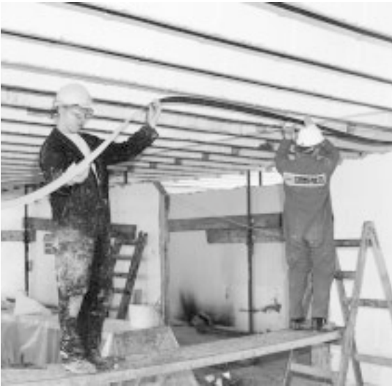
Figure 11.3 Positioning an 11.0m laminate to underside of rib.
