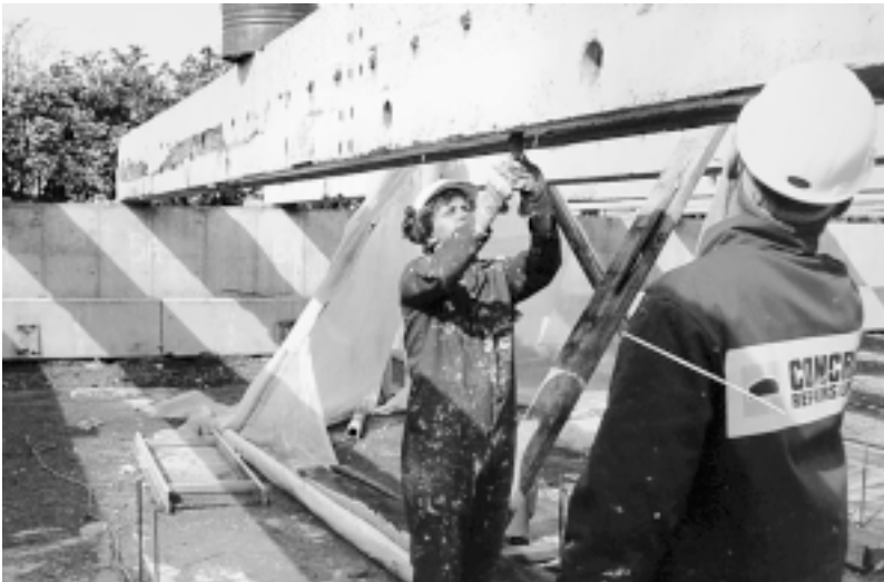
Figure 10.4 Using a hard rubber roller to squeeze out excess adhesive and ensure firm adhesion.
