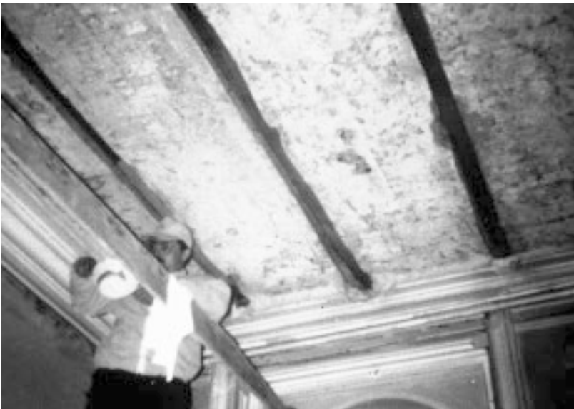
Figure 11.31 Application of CarboDur laminates.
