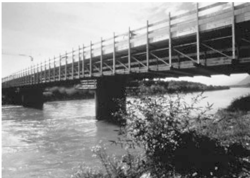
Figure 11.5 General view of Oberriet bridge.
