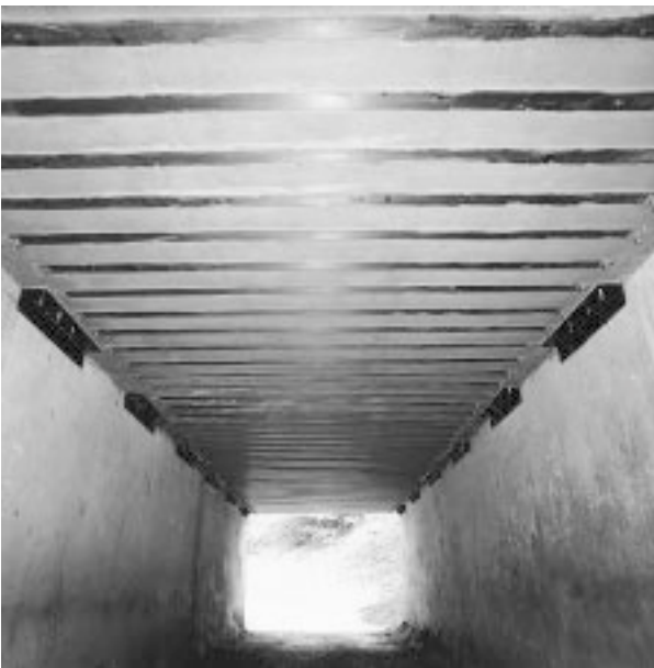
Figure 11.27 Completed bonding operation of underpass, Great Missenden.
