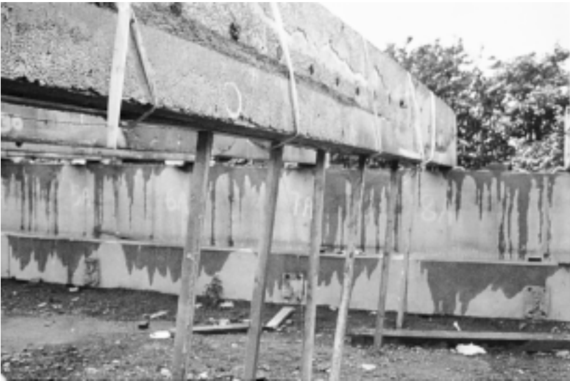
Figure 10.11 Props and bearer beams installed to prestressed plate.
