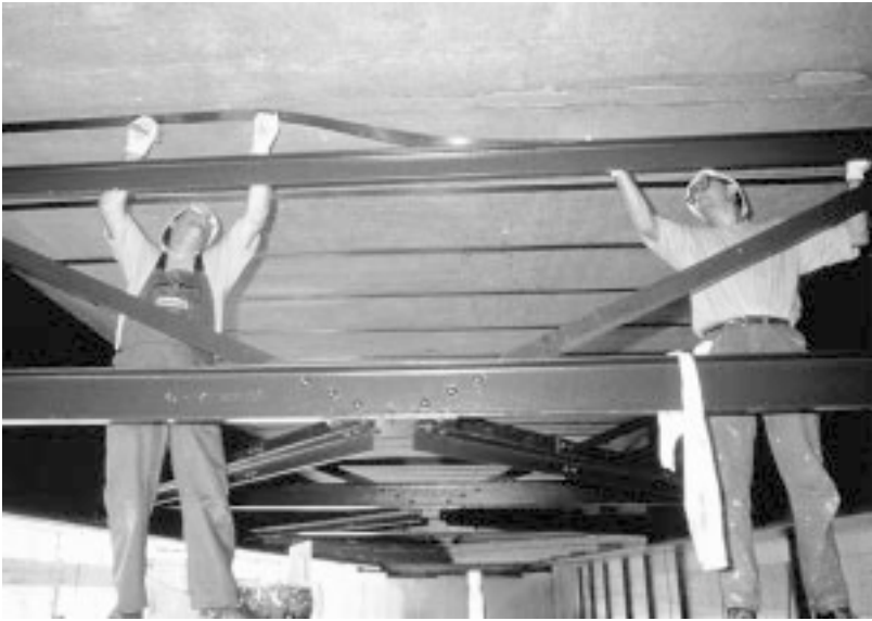
Figure 11.10 Installation of CarboDur laminate.
