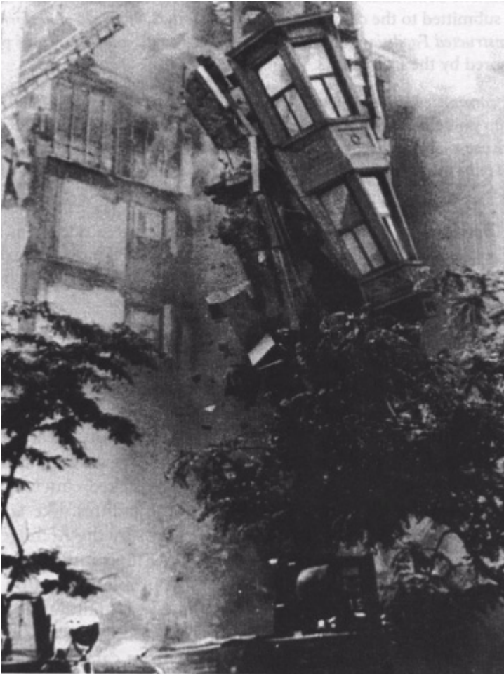
Figure 8.1 The historic Hotel Vendome in Boston, Massachusetts, collapsed suddenly during a fire.
