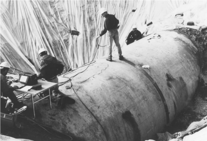
Figure 8.14 Impact-echo testing of deteriorated concrete pipe detects internal cracks and delaminations.
