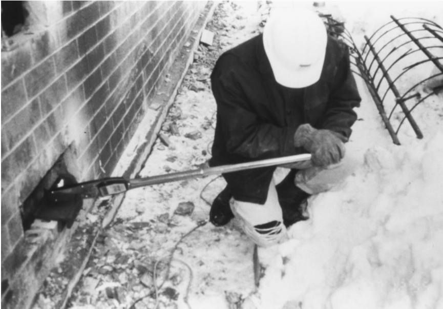
Figure 8.15 Bond-wrench testing on in situ brick masonry.
