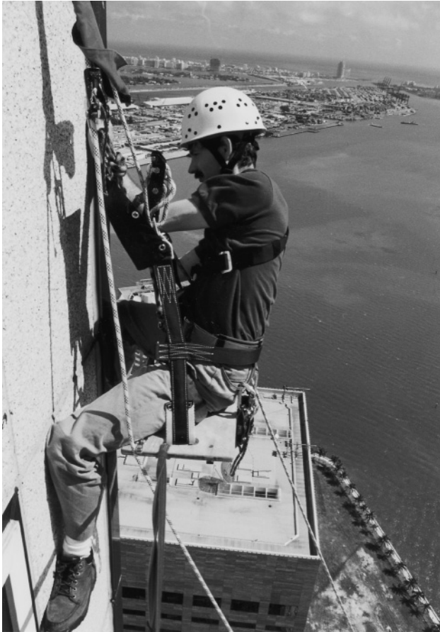
Figure 8.9 Investigating engineer gets the facts first hand through industrial rope access.
