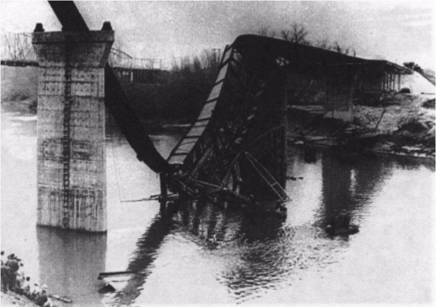
Figure 8.2 Collapse of Brazos River Bridge, Texas.
