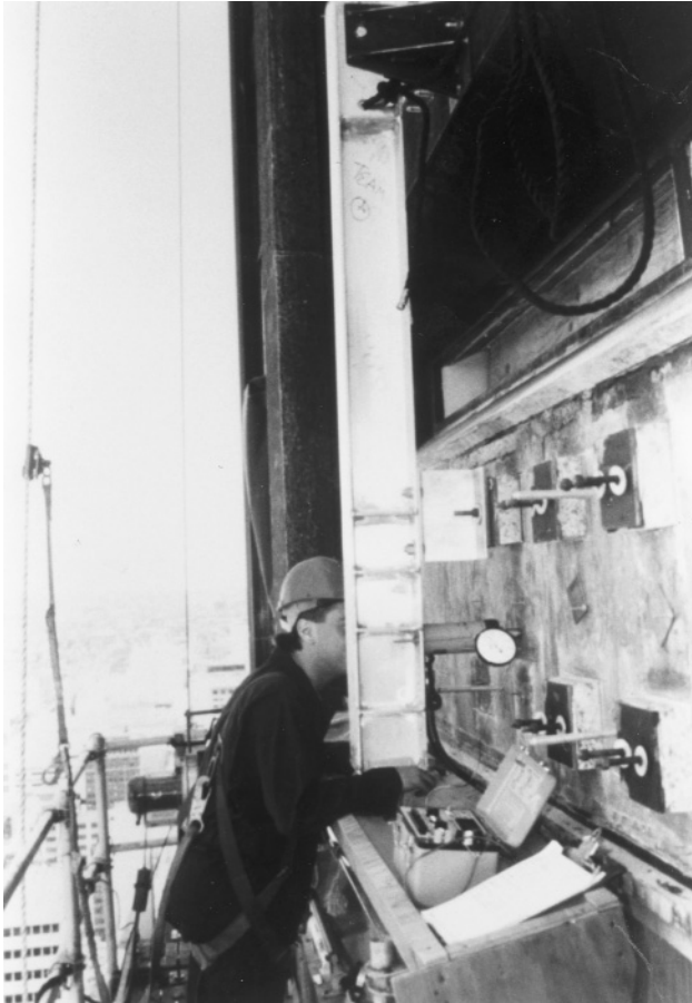
Figure 8.11 In-field pull-out tests on stone anchors.
