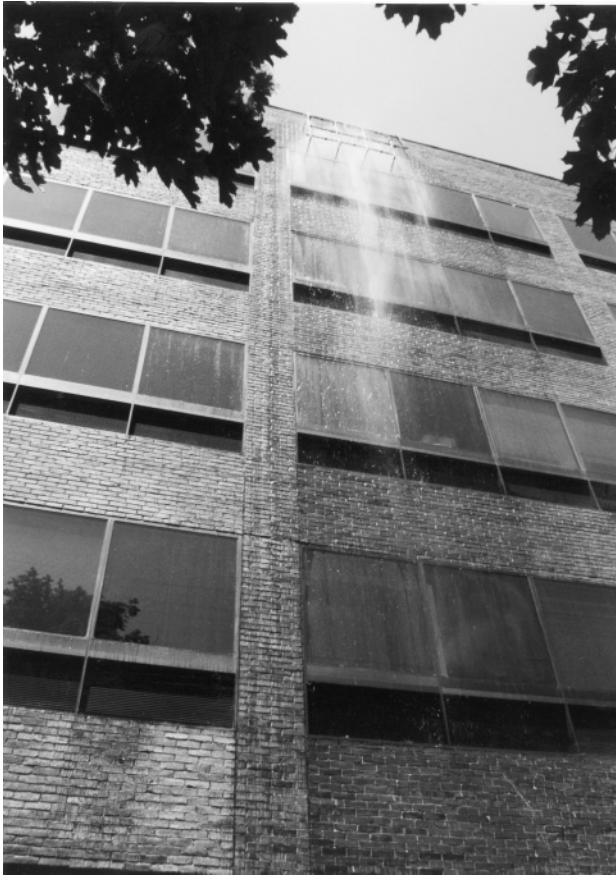
Figure 8.16 In-field water test on building cladding.
